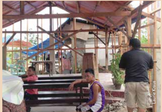
Outside Palo, near Tacloban, a farming village church of the UCCP begins to rebuild with coco wood, a plentiful building resource now that the area's coconut trees and plantations have been destroyed by Haiyan. This important crop tree will have to be replanted. With no coconut fruit yield expected for 5-7 years, the farming economy, dependent on coconut and rice, will be severely challenged
